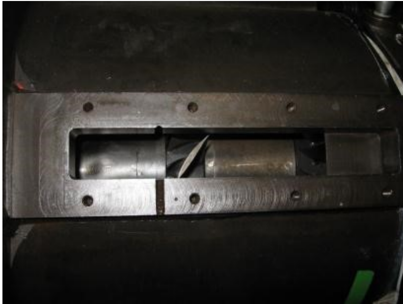
Figure A7 View of an instrumentation access window.
