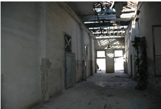
Fig. 4.3.13: Corridor on the first floor
