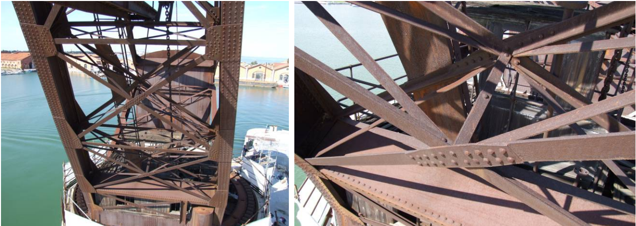
Fig. 5.3.15: The bracing beams stiffening the two main struts
