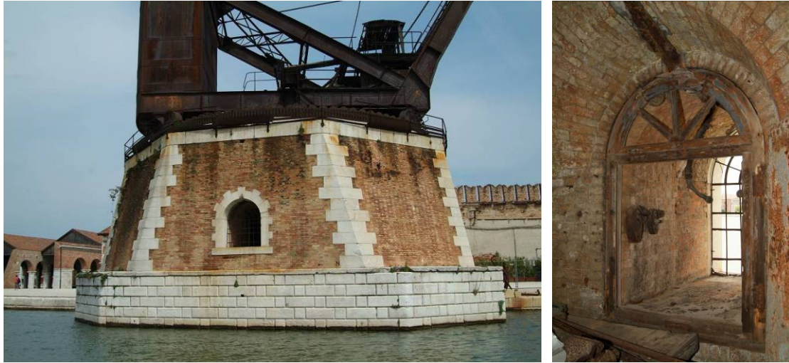
Fig. 5.8.24: View of the basement and of the wall's thickness
