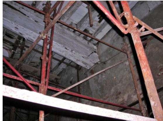
Fig. 4.4.16: End of the beam supported by masonry corbel
