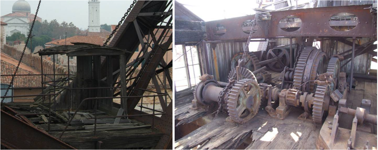
Fig. 5.3.26: The cabin and the gears needed for the crane's operation
