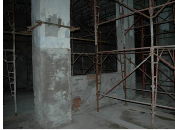
Fig. 4.4.70: Base of the pillar 15, connected with the pillar 14
