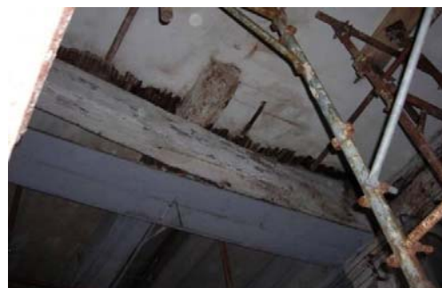
Fig. 4.4.31: Element supporting the purlins
