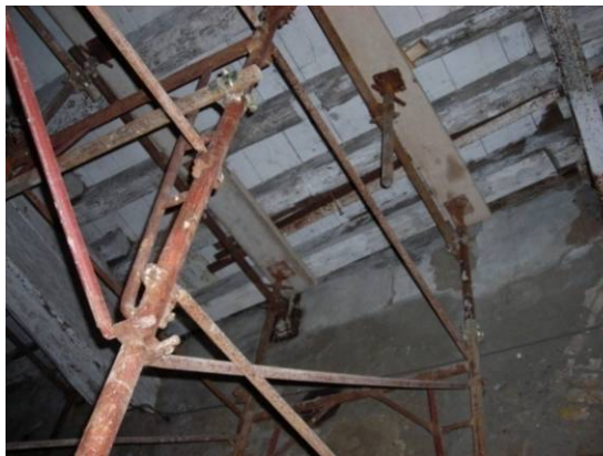
Fig. 4.4.50: Two span beam. View of the iron I-Beam
