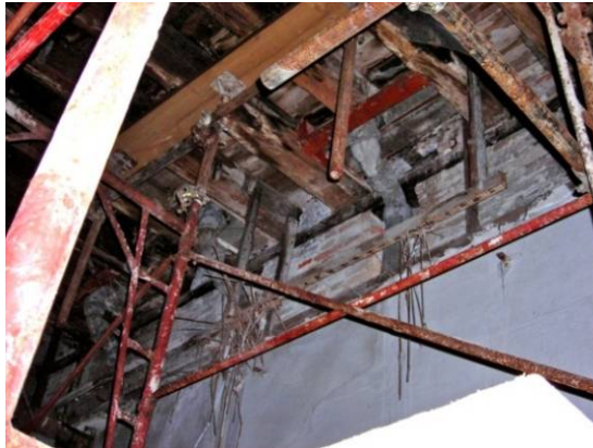
Fig. 4.4.40: Wooden joist used in the connection beam-wall
