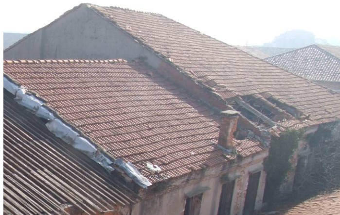
Fig. 4.4.127: View of the roof of the areas B and C
