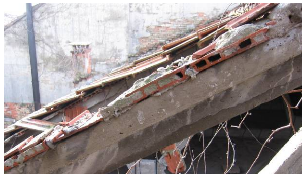
Fig. 4.4.114: “Perret” tiles leans in a strut
