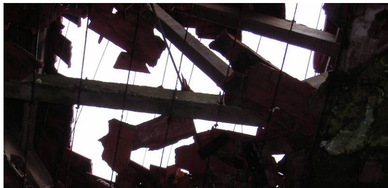
Fig. 4.4.125: View of the beam system of the area C
