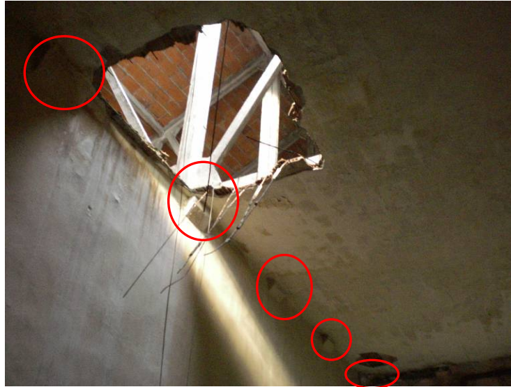
Fig. 4.4.120: support corbels of the trusses
