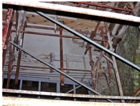
Fig. 4.4.8: Lateral wooden tackling and stirrups at the end beam
