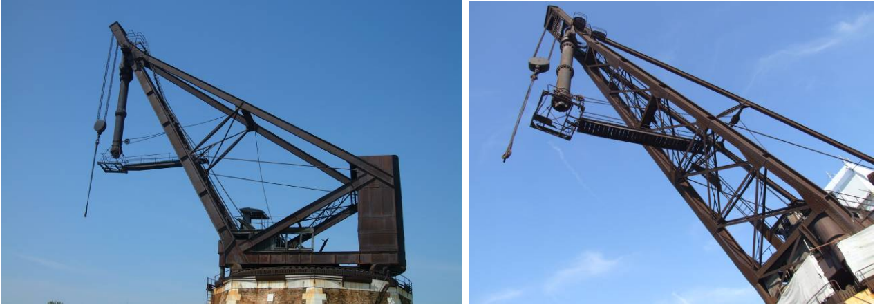
Fig. 5.3.12: The reticular boom showing its lattice pyramid shape
