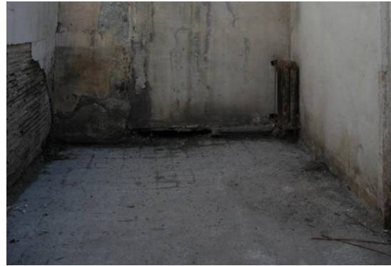
Fig. 4.4.35: Depression of the floor
