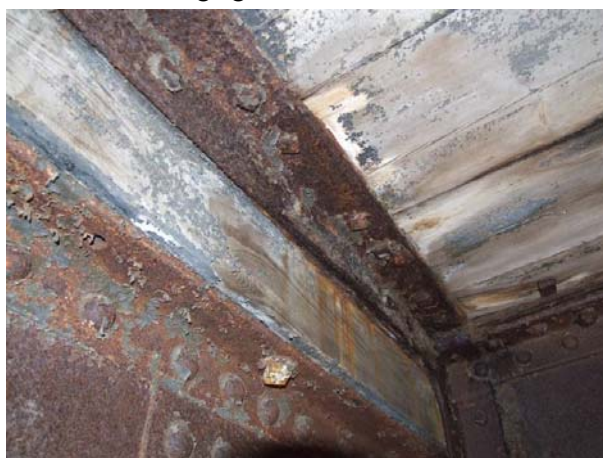
Fig. 5.8.23: Beam detail that needs cleaning and processing
