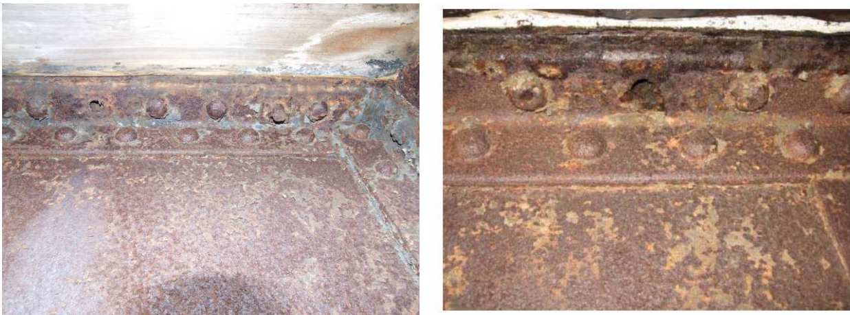
Fig. 5.4.45: Missing rivets
