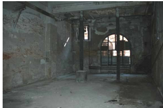
Fig. 4.3.11: I-Beams supporting brick vaults
