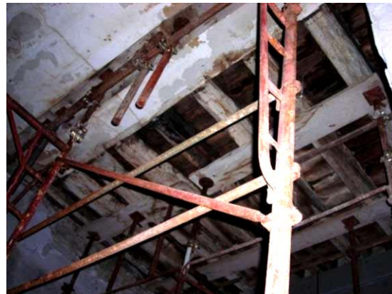
Fig. 4.4.45: Floor wooden frame
