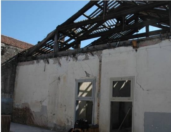
Fig. 4.3.17: Portion of the wooden partition covered by secondary beams nailed and plastered
