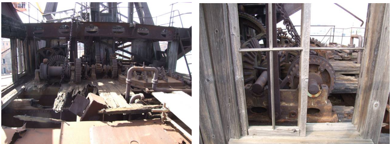
Fig. 5.8.21: Current condition of the engine room
