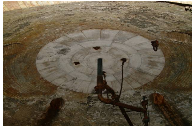
Fig. 5.3.3: The stone ashlar on the top of the basement
