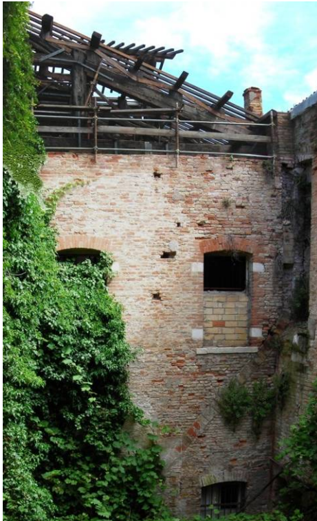
Fig. 4.3.15: North façade of the internal courtyard of the building
