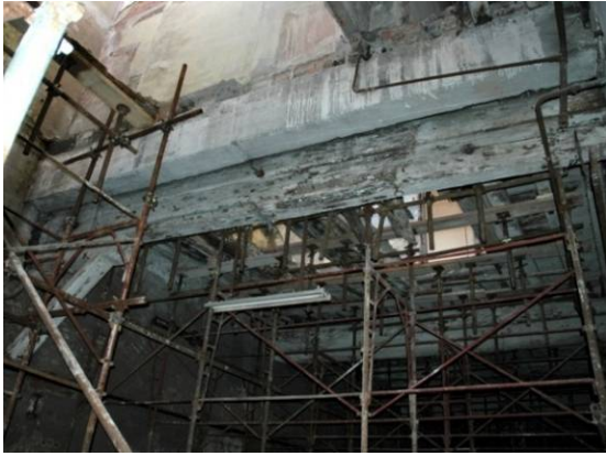
Fig. 4.4.19: Reinforced concrete beam and wooden beams placed side by side
