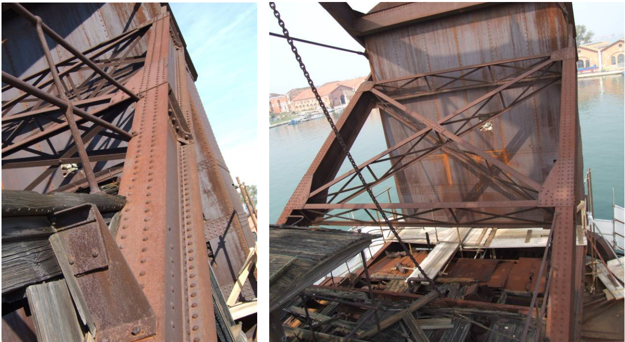
Fig. 5.3.13: The lower strut and the stiffening system
