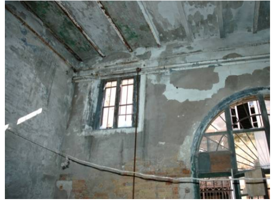
Fig. 4.3.20: Floor in iron beams and brick vaults
