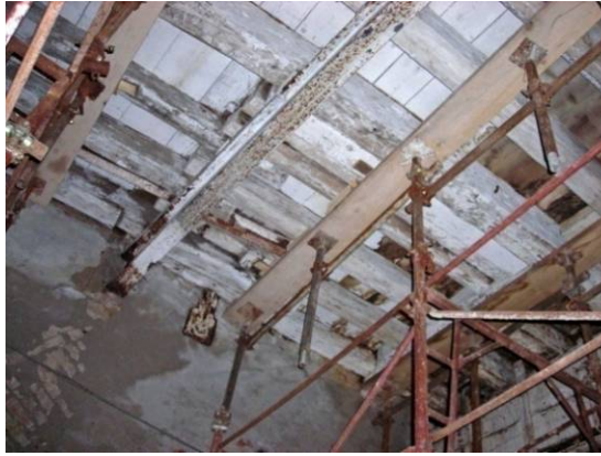
Fig. 4.4.47: Two span purlin rests on supporting wooden beam and on beam 5
