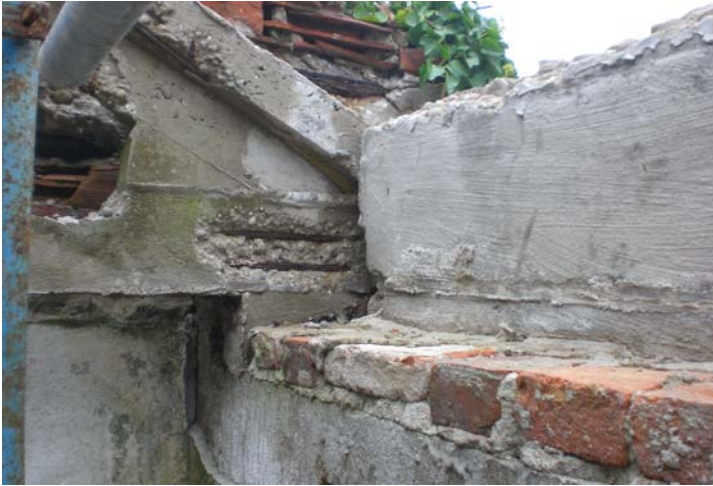
Fig. 4.4.96: Detail of the curb
