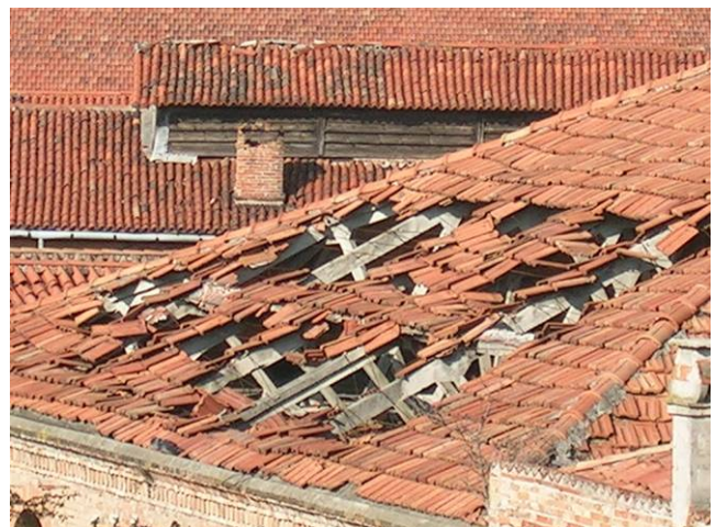
Fig. 4.4.131: View of the reinforced concrete beams that form the pavilion roof
