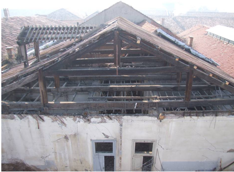
Fig. 4.4.75: View of the wooden trusses of the area A
