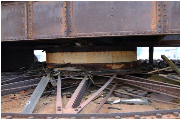
Fig. 5.3.3: The stone ashlar on the top of the basement
