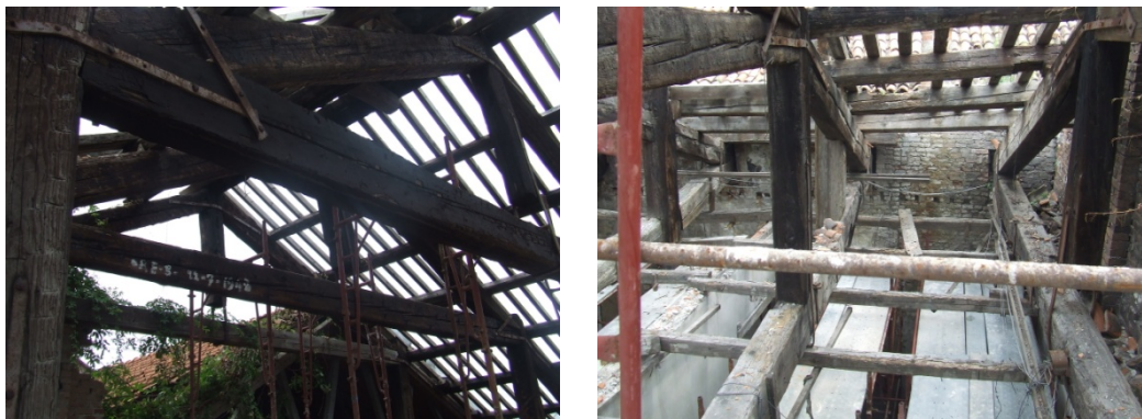
Fig. 4.6.12: Wooden trusses before the intervention of conservation
