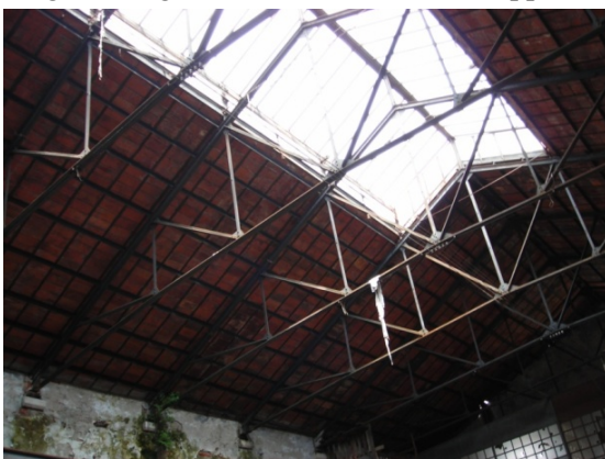
Fig. 4.6.3: Internal view of the maritime warehouse roofing: “English” trusses and skylight
