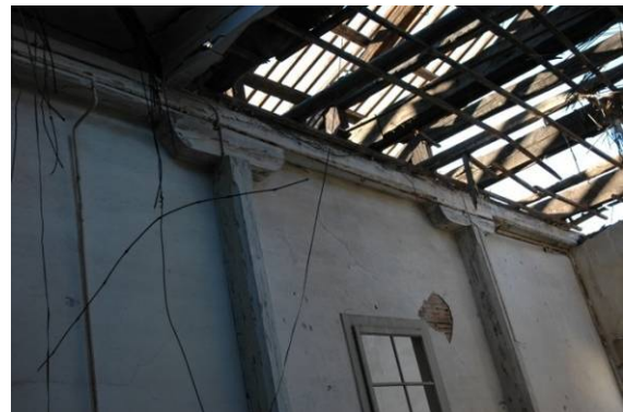
Fig. 4.3.14: Wooden pillars with barbican supporting the wooden beam
