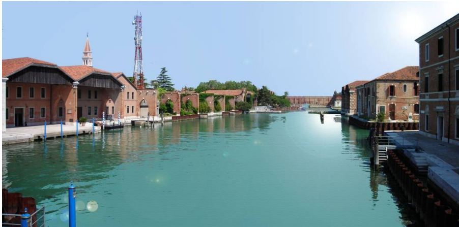
Fig. 3.6.1: View of “Darsena Vecchia” and of the "Galeazze" channel
