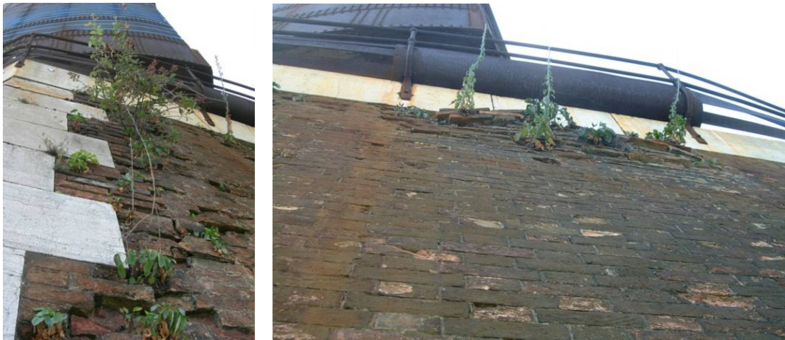
Fig. 5.4.29: Masonry's disconnections
