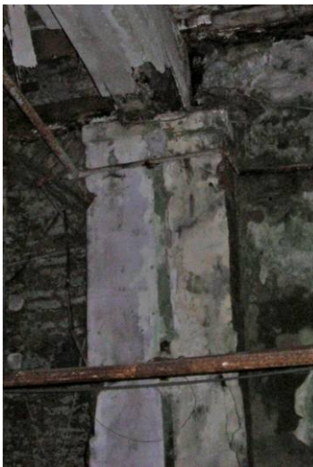
Fig. 4.4.60: Capital at the end of the pillar 4
