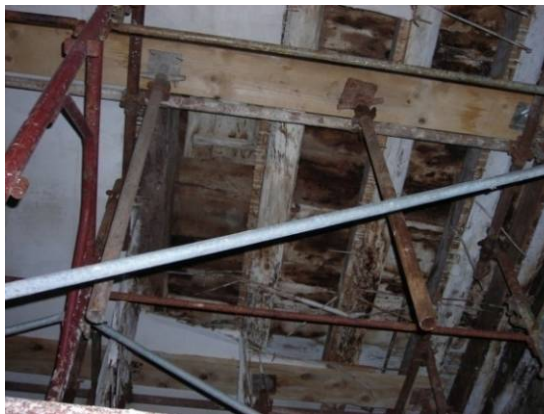
Fig. 4.4.32: Purlins and wooden plank
