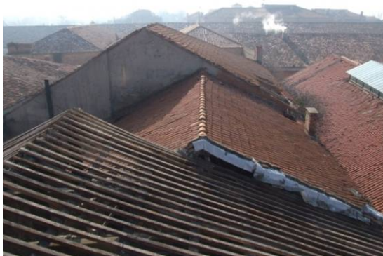
Fig. 4.3.26: Different heights of the roof of the "Sala Maggiore"
