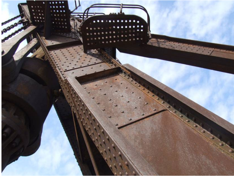
Fig. 5.3.16: Upper part of the main struts
