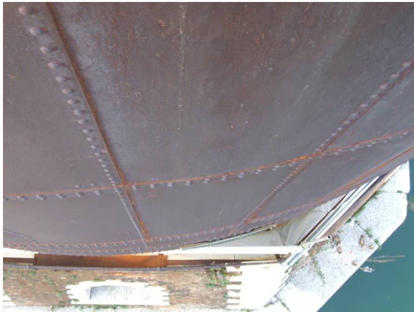
Fig. 5.3.21: The external strengthening system of the counterweight
