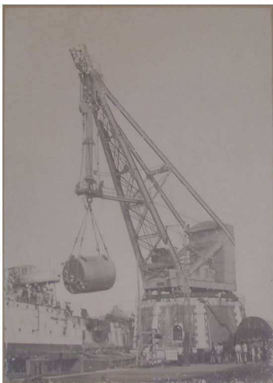
Fig. 5.2.7: The Armstrong crane during the installation of a boiler on a ship (Bovolenta, 2005)
