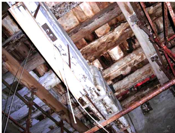
Fig. 4.4.43: Purlins supported by the main beam 5
