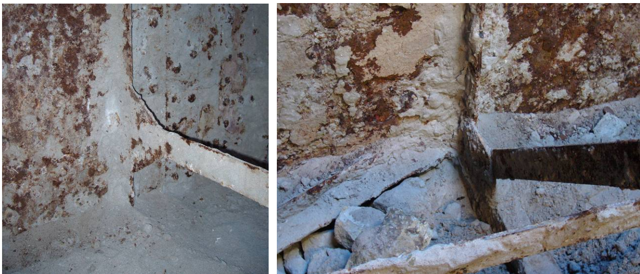
Fig. 5.7.13: connection node between horizontal and vertical elements
