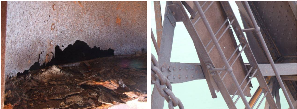
Fig. 5.4.43: Sheets corrosion
