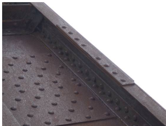
Fig. 5.4.4: Detail of the rivets pitch
