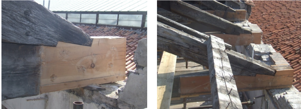
Fig. 4.6.15: Reconstruction of the tie beam-strut joint
