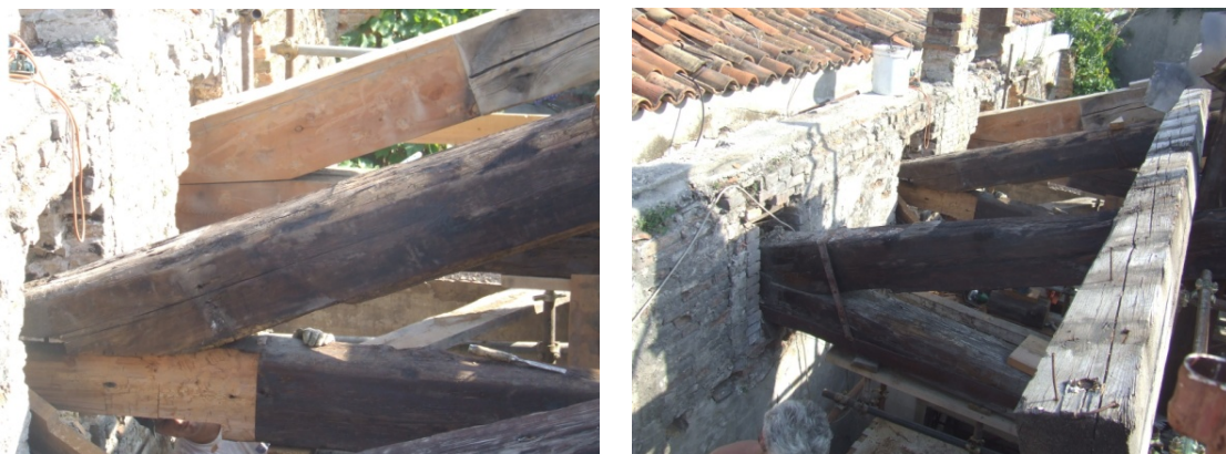
Fig. 4.6.14: Resection of the deteriorated sections
