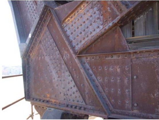
Fig. 5.6.10: Detail, node of the crane where three trusses converge
