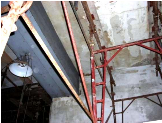
Fig. 4.4.44: False ceiling of the first floor
