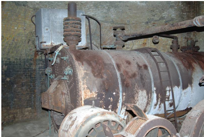
Fig. 5.4.44: Engine room degradation
