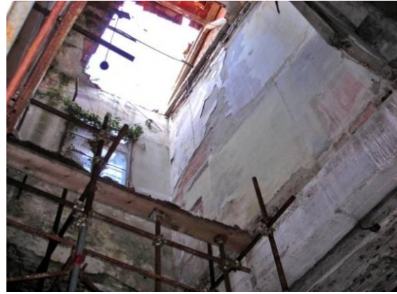
Fig. 4.4.20: Reinforced concrete beam
