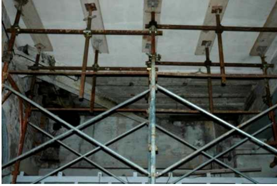
Fig. 4.4.22: Purlins near the wall
