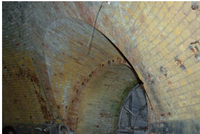
Fig. 5.4.20: Detail of masonry in the intrados of the vault
