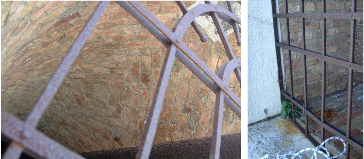
Fig. 5.4.19: Detail of internal masonry
