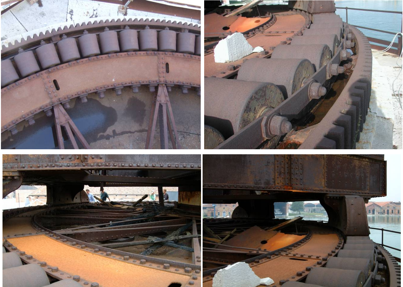
Fig. 5.3.7: Ring gear, rollers and sheet ring of steel-structured body
