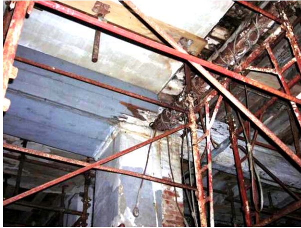
Fig. 4.4.42: Floor frame hidden among the false ceiling
