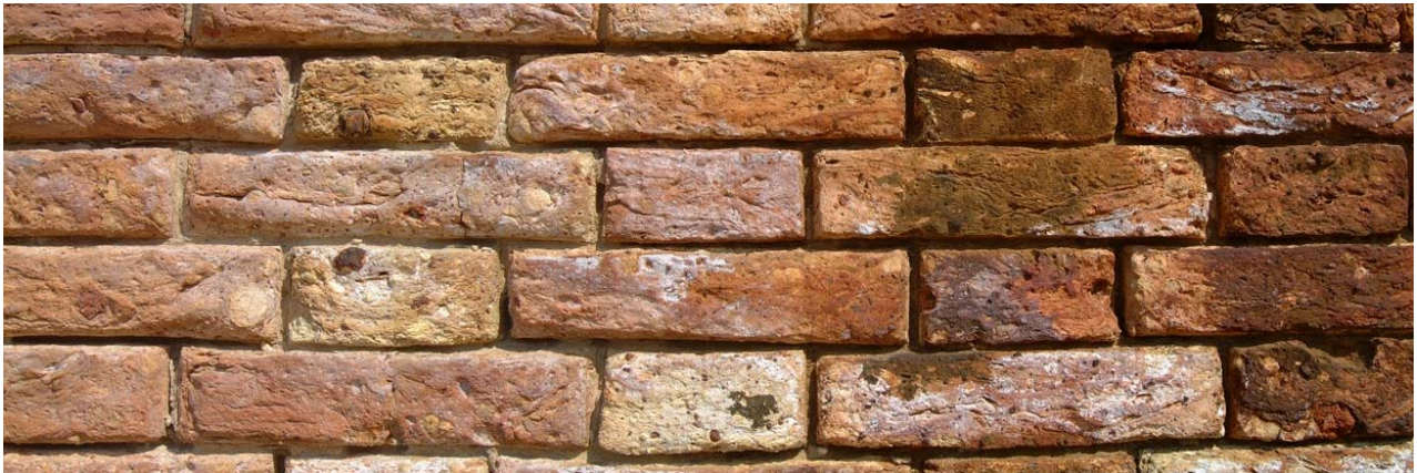
Fig. 5.4.18: Detail of external masonry
