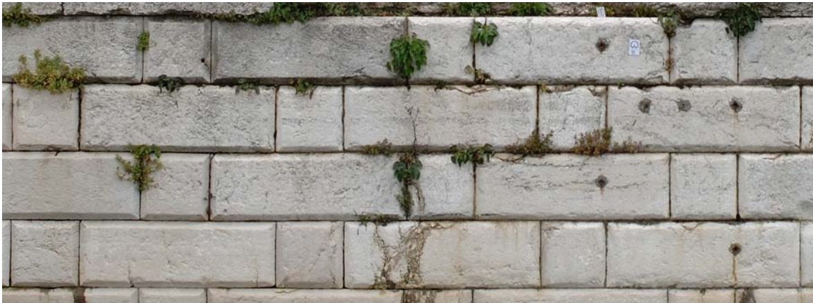
Fig. 5.4.14: Detail of the Istrian stone basement
