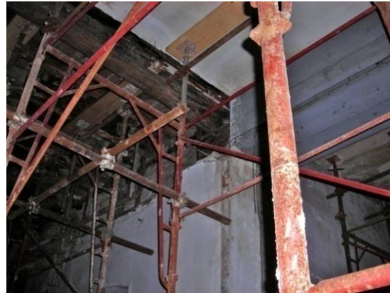
Fig. 4.4.41: Beam placed in the pillar 10 and in the main beam 4
