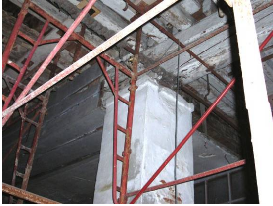
Fig. 4.4.69: Superior end of the pillar, made by a slab of stone
