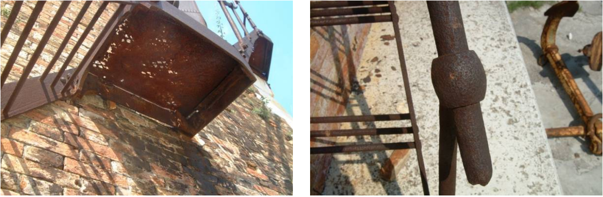
Fig. 5.4.37: Iron stairs to reach the upper part of the basement
