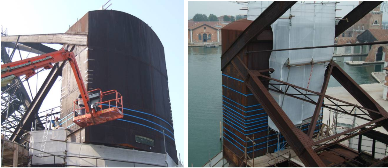
Fig. 5.7.7: Safety intervention with 12 temporary reinforcement rings
