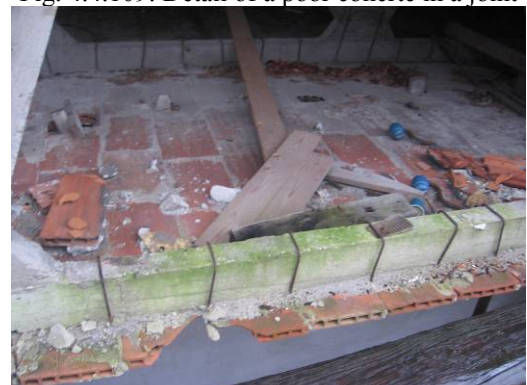
Fig. 4.4.111: Detail of a biological patina in a strut
