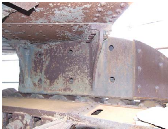
Fig. 5.6.8: Detail, connection sliding block – balance weight caisson
