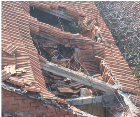
Fig. 4.4.129: View of the trusses C1 and C2
