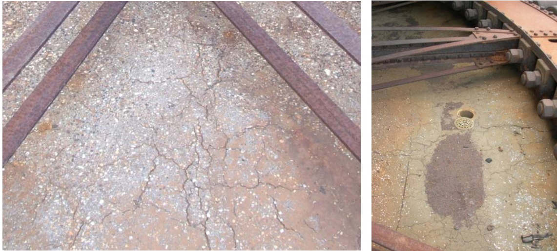
Fig. 5.4.21: Detail of the concrete layer
