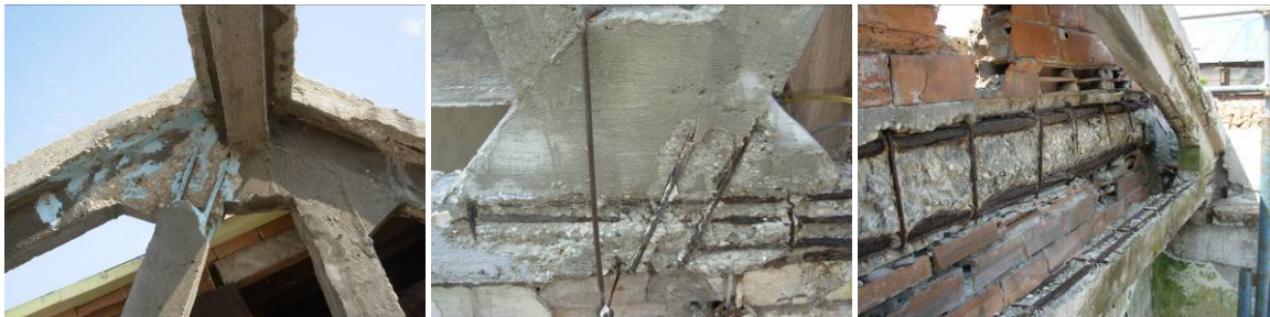
Fig. 4.4.102: Details of the actual conditions of the reinforced concrete trusses
