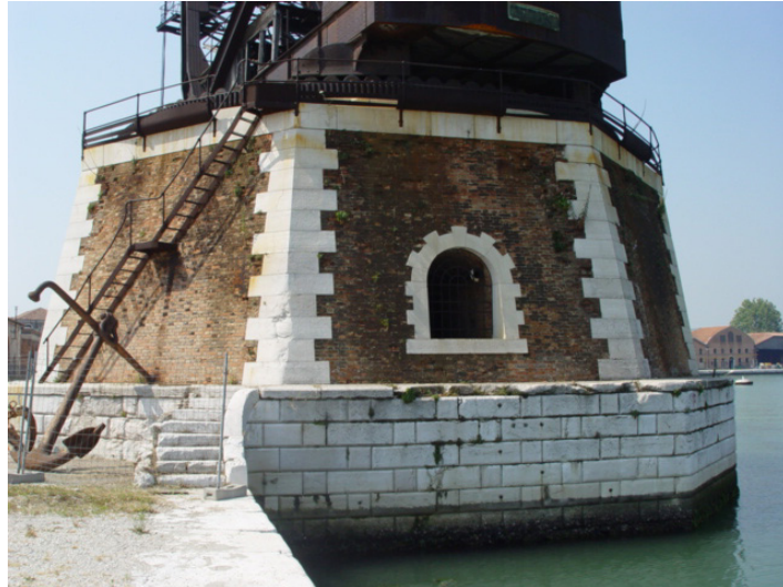
Fig. 5.3.2: The masonry basement of the crane
