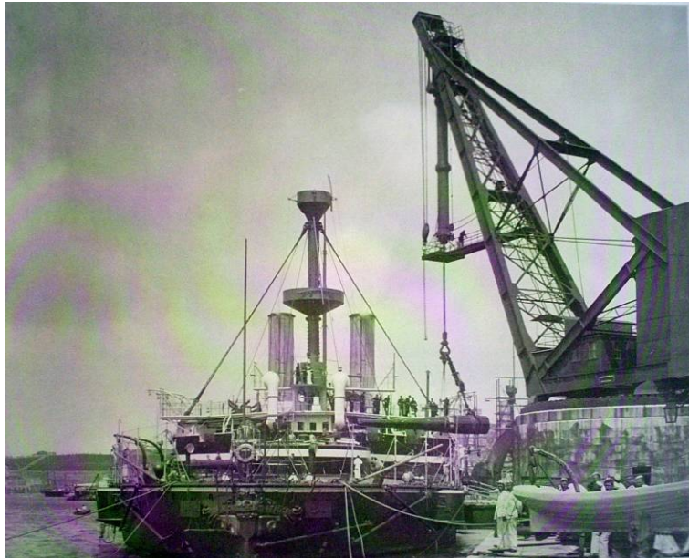
Fig. 5.2.3: The crane of Malta during the loading of a 67tons cannon on the ship Trafalgar, 1896 (B. Warlow e R.Ellis, 1989)
