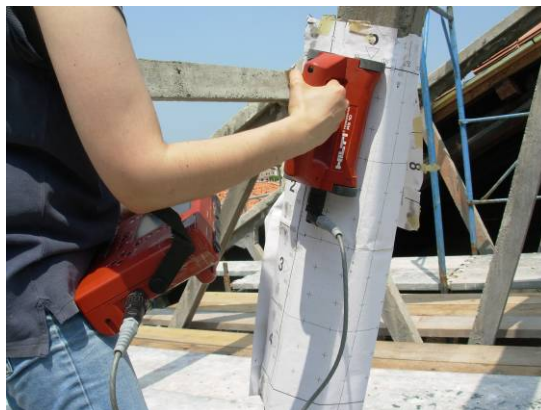
Fig. 4.4.100: Detail of the test with electromagnetic cover meter
