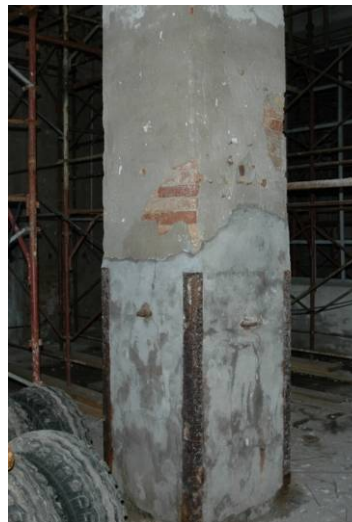
Fig. 4.4.61: Metallic sections at the edges of the pillar 2
