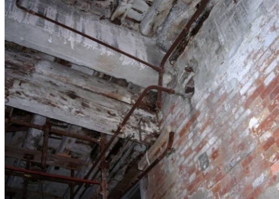
Fig. 4.4.18: Slab of stone for the connection beam-wall
