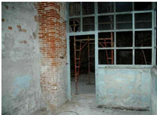
Fig. 4.4.71: Masonry pillar against the wall
