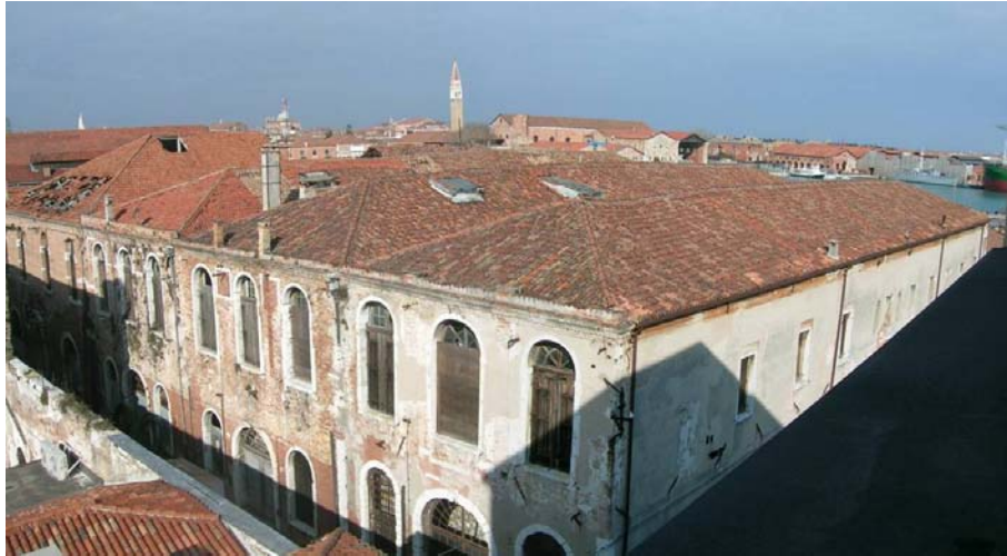
Fig. 4.2.9: South-east view of the complex of the “ Sale d'Armi Nord ”
