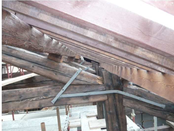
Fig. 4.6.17: Restored joints of the trusses of the area A
