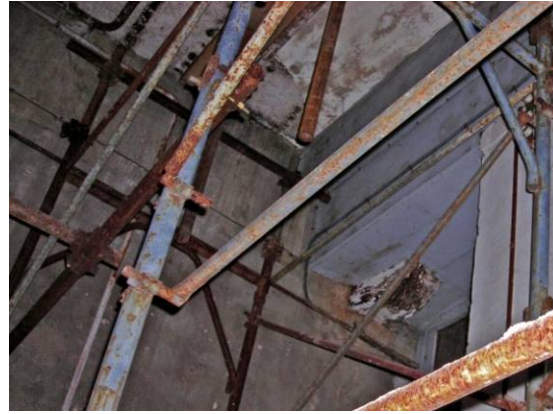
Fig. 4.4.29: Main beam 2 on which rest the purlins
