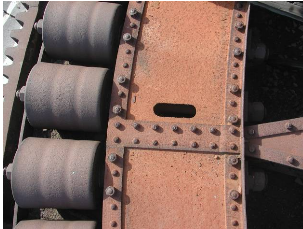
Fig. 5.4.47: Ware due to rollers rubbing
