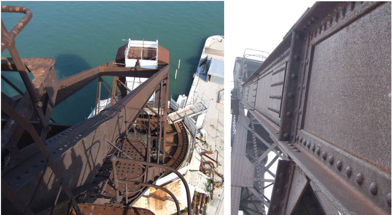
Fig. 5.3.17: Main tie beams
