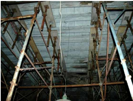
Fig. 4.4.38: Secondary frame of the floor
