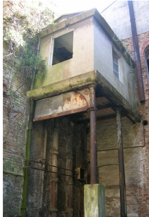
Fig. 4.3.16: Construction projecting supported by cast iron columns
