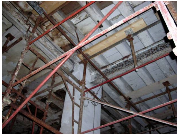
Fig. 4.4.68: Iron beam restrained at the pillar
