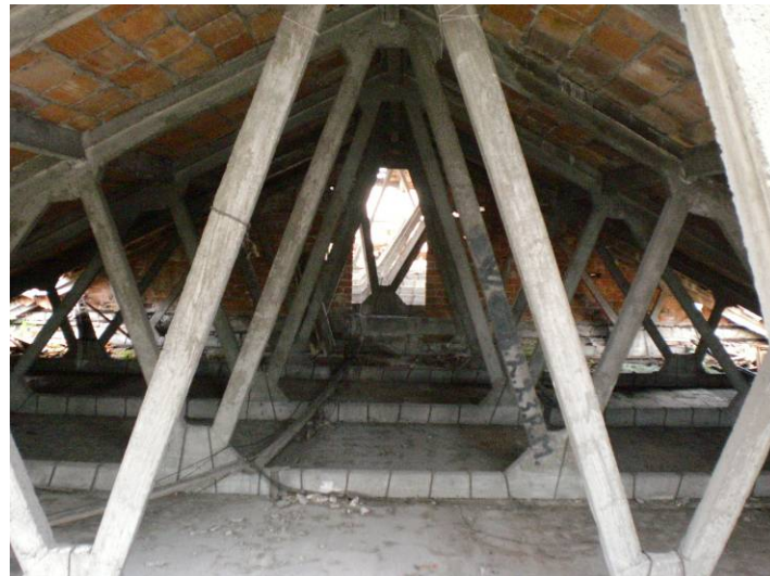
Fig. 4.4.87: View of the reinforced concrete trusses of the zone B
