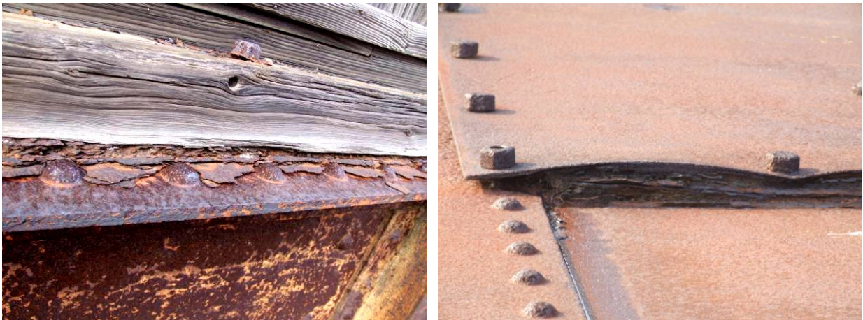
Fig. 5.4.40: Examples of puddle iron parts exfoliation
