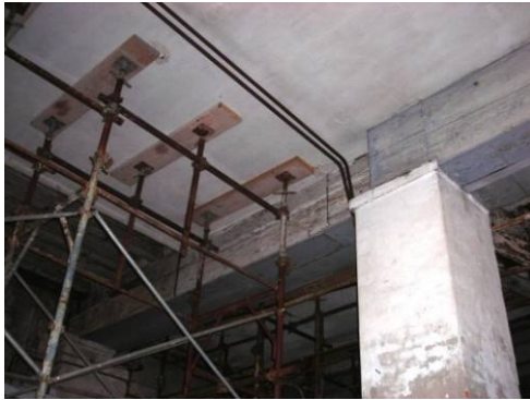
Fig. 4.4.5: First span: connection between two wooden beams
