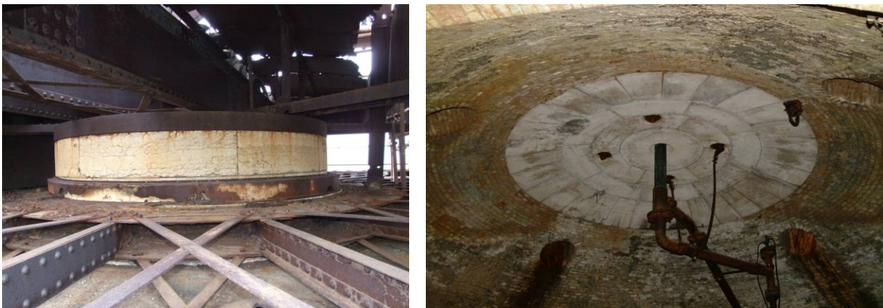
Fig. 5.4.16: Details of external and internal ashlar
