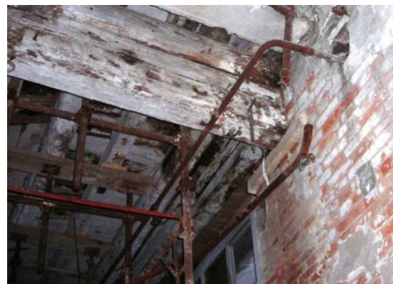
Fig. 4.4.72: Slab of stone at the end of the pillar
