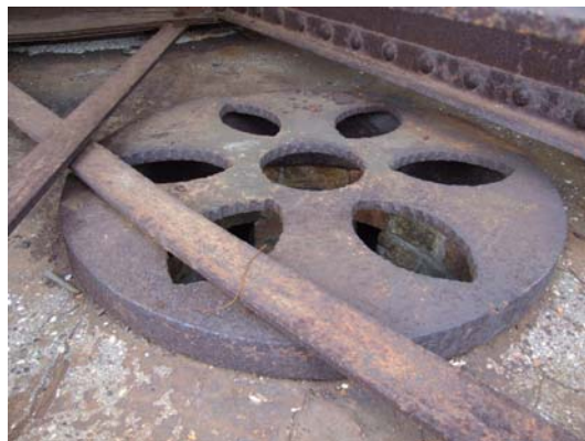
Fig. 5.8.10: Detail, water drains
