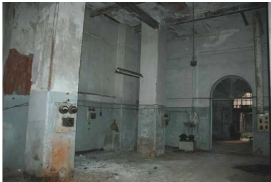
Fig. 4.3.10: Plastered masonry pillars
