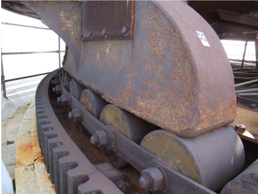
Fig. 5.8.15: Detail of the rollers upon which one of the four sliding blocks lies
