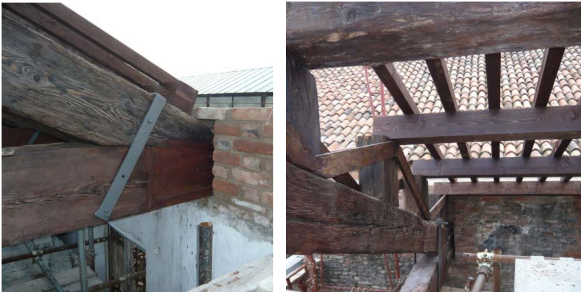
Fig. 4.6.18: Restoration intervention in the end of the tie beam
