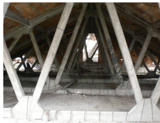
Fig. 4.3.27: Reinforced concrete trusses and "Perret" false ceiling
