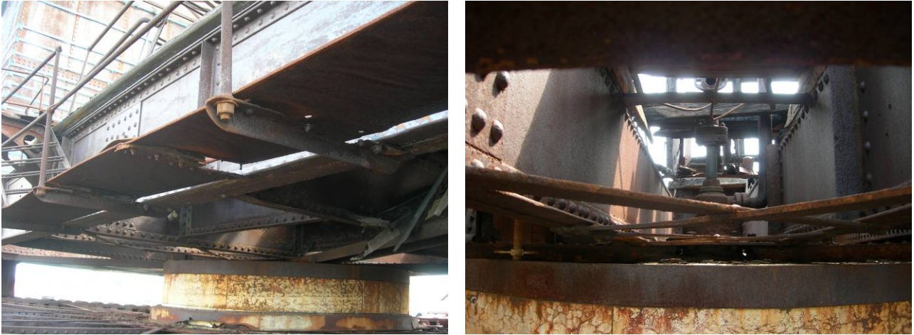
Fig. 5.3.10: The reinforcements beams of the horizontal frame
