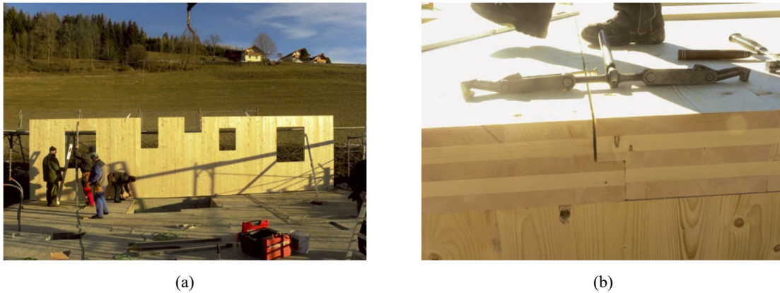
Fig. 2.14 – Assembling of large horizontal panels [2.63]: (a) façade panel; (b) floor.
