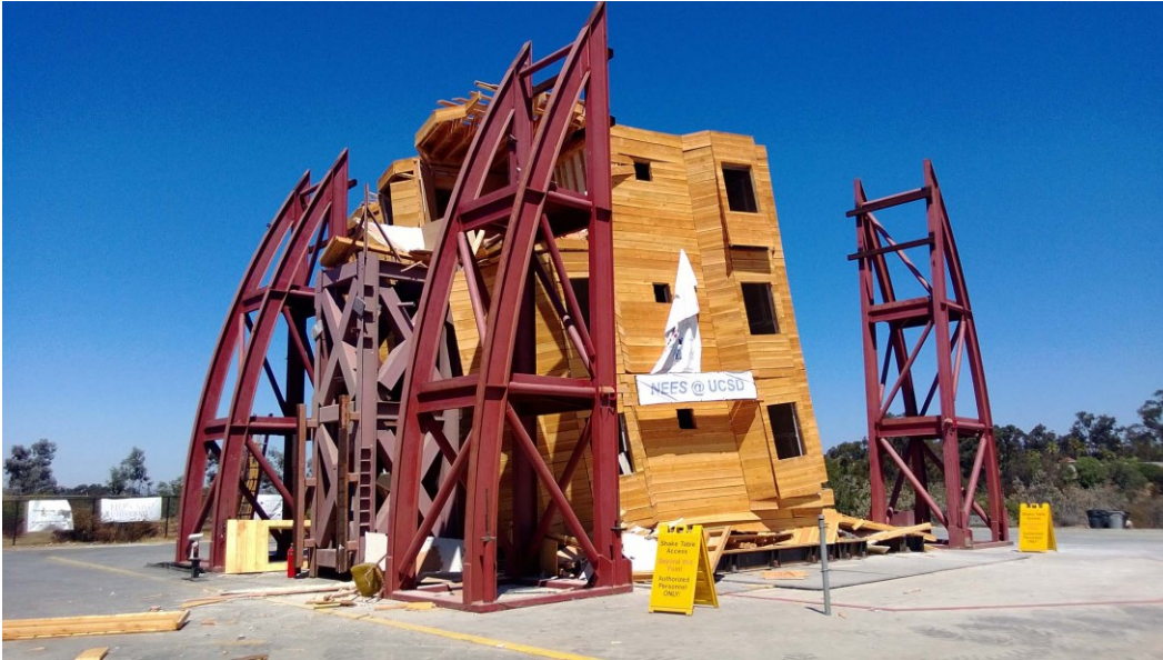
Fig. 2.26 – NEES-Soft project. Collapse of a wood-frame building due to “soft-storey” mechanism. [2.71]
