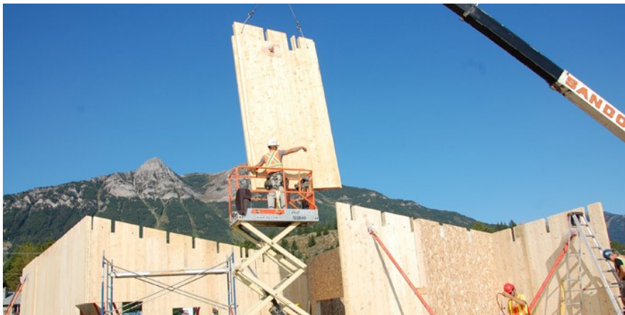
Fig. 2.15 – Assembling of small jointed panels [2.64].
