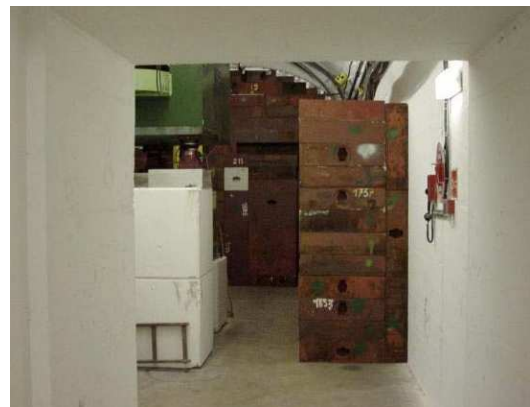
(b) View of the iron shielding placed after the sweeping magnet.
