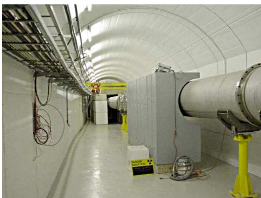
(a) Additional concrete shielding placed after the spallation target zone.
