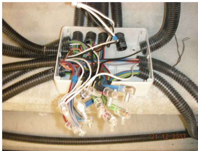
Figure 8-89 Power and Bus Connections
