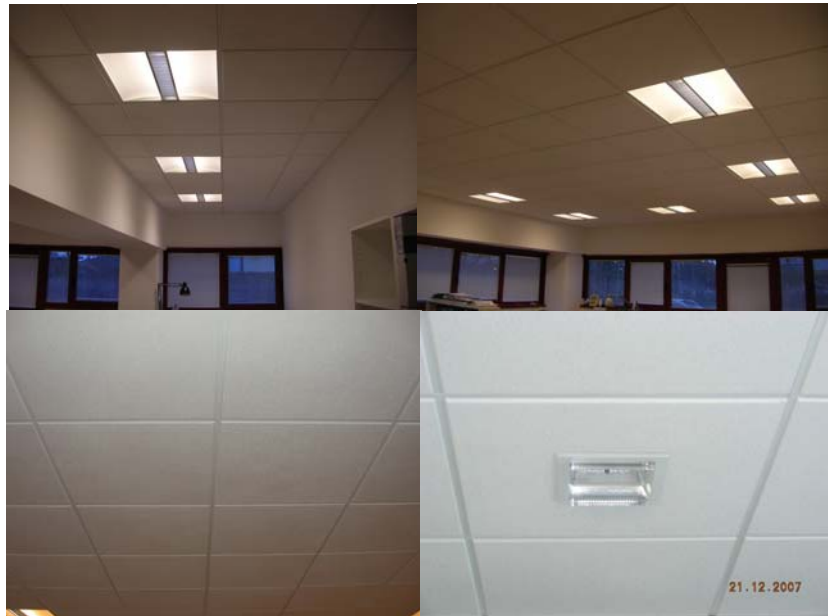
Figure 8-95 New luminaires and new plaster ceiling
