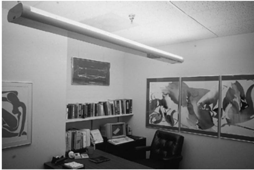
Figure 7-9. Pendant luminaires are commonly used to provide indirect illumination.
