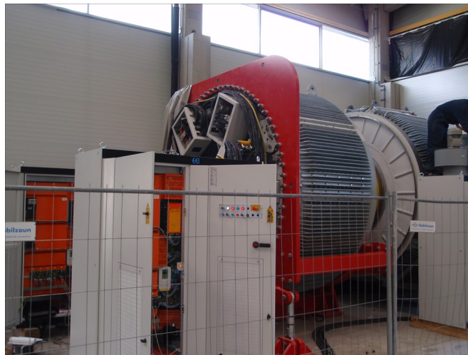
Figure 2.24: B2B test bench in Telfs
