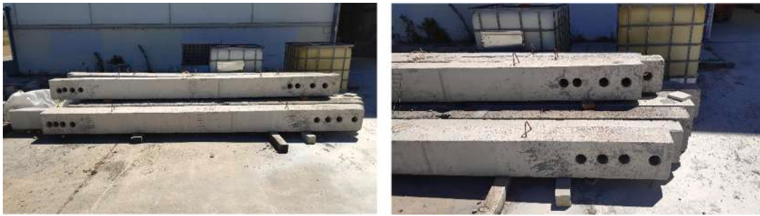
Fig. 3. Location of core drilling in the full beams (left) and detail of the ends of the beams (right).
