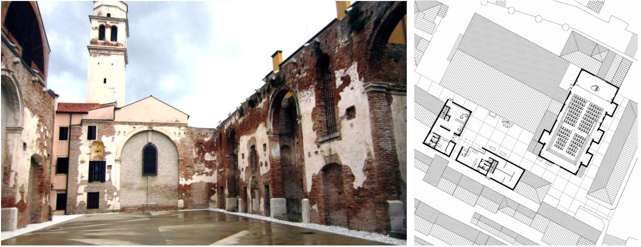
Figure 11. Remains of the eighteenth-century church. Internal view towards the apse.
