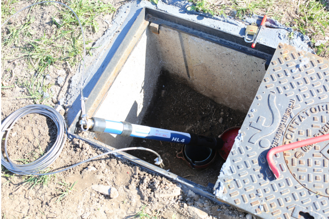
Figure 2.10: Installation of the Hydrolab HL4 multi-parametric probe.
