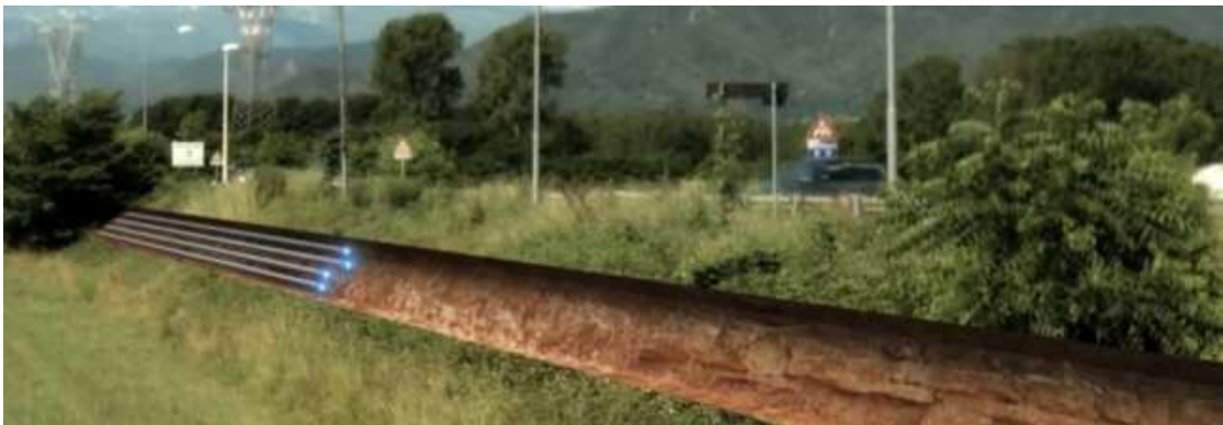
Figure 1.39: Cable trench close to the highway
