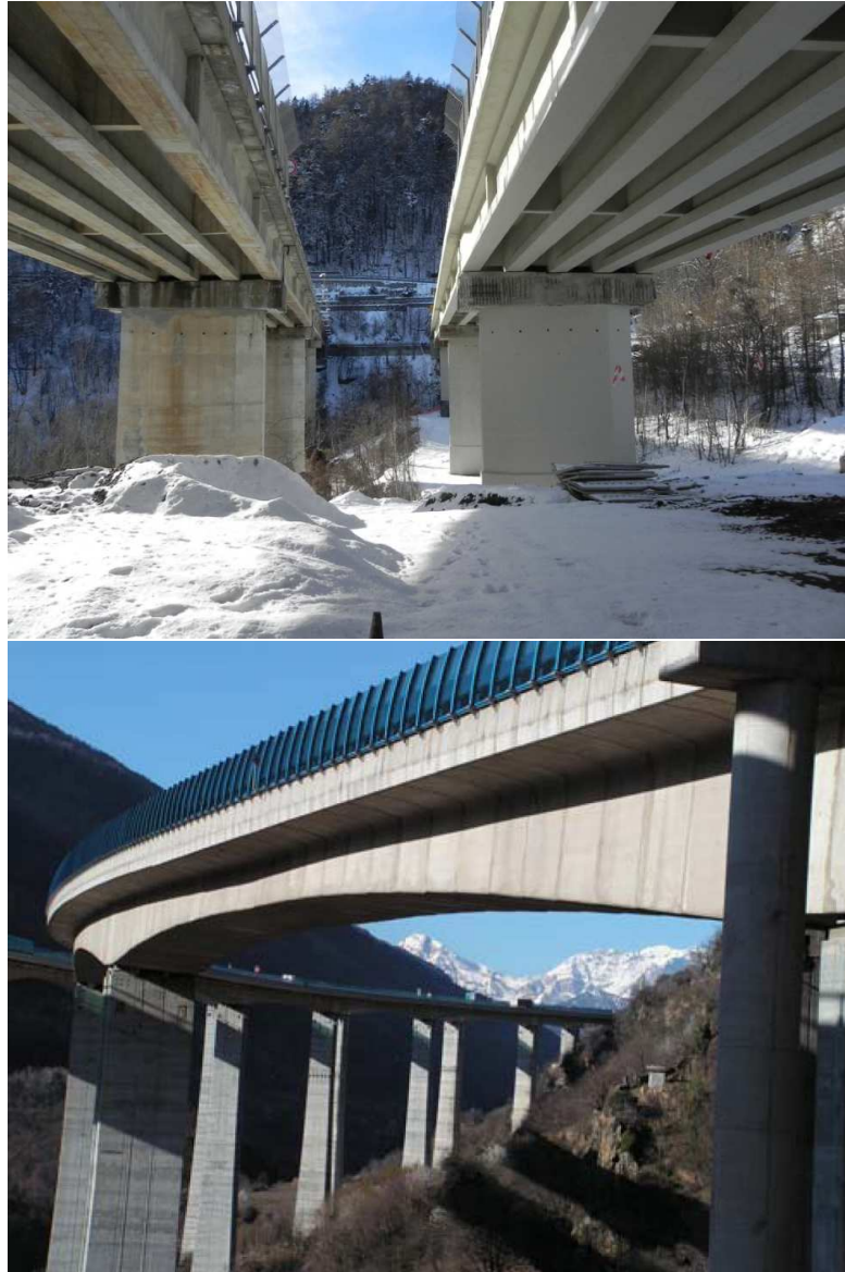
Figure 1.42: Viaducts of the A32 Highway
