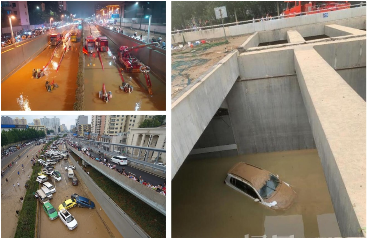
Figure 1-10 The waterlogging in urban lowlands (tunnels and culverts). (Source: China Daily)
