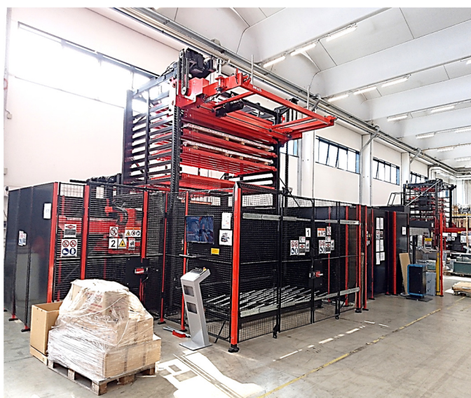
Figure 7. Part of the newly installed laser-cut machine (Case 2—own research).
